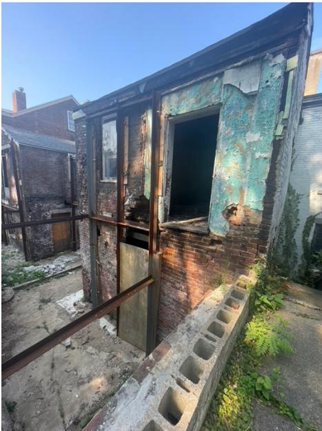
When concrete work was being done, contractors expressed a concern about the structural integrity of the rear façade of both halves of the building, so they could not do floor work in the rear (third) room of each. We then had the rear façade reinforced with temporary steel bracing, and rear room paving was postponed. The bracing will be removed when masonry work is completed and the rear walls are stable on their own.
