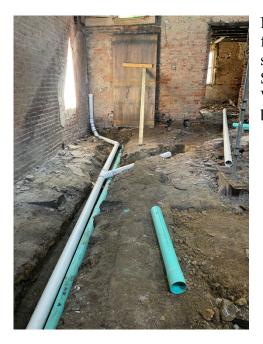
Now that warm weather is here, construction is moving forward. The photo on the left shows the new sanitary and storm sewer lines in the 724 Main half of the duplex. Similar lines are now in place in the other half, as well. Water lines have also been run to both halves. The photo below shows exterior excavation work.
