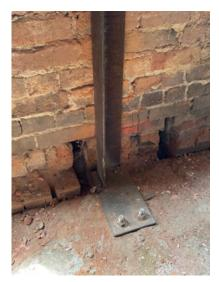
Steel beams have now been installed along the interior walls on the front and alley sides of the duplex – one beam on the front of each of 722 and 724 Main and five beams along the alley
