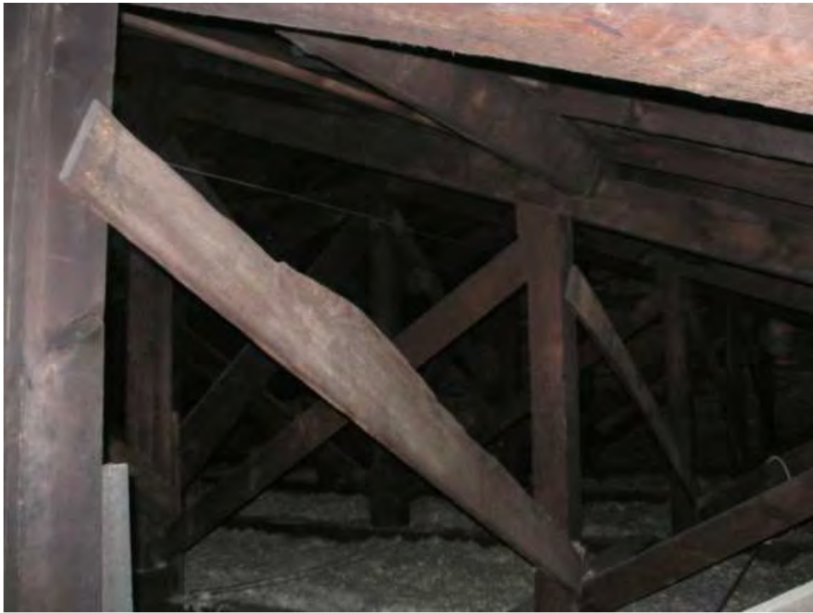
Photo 11. View of Roof Truss Framing and Cross Bracing in Attic
