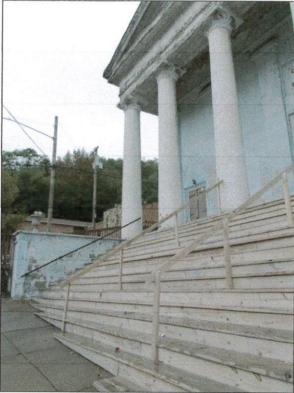
Wood Clad Stone Front Stairs
