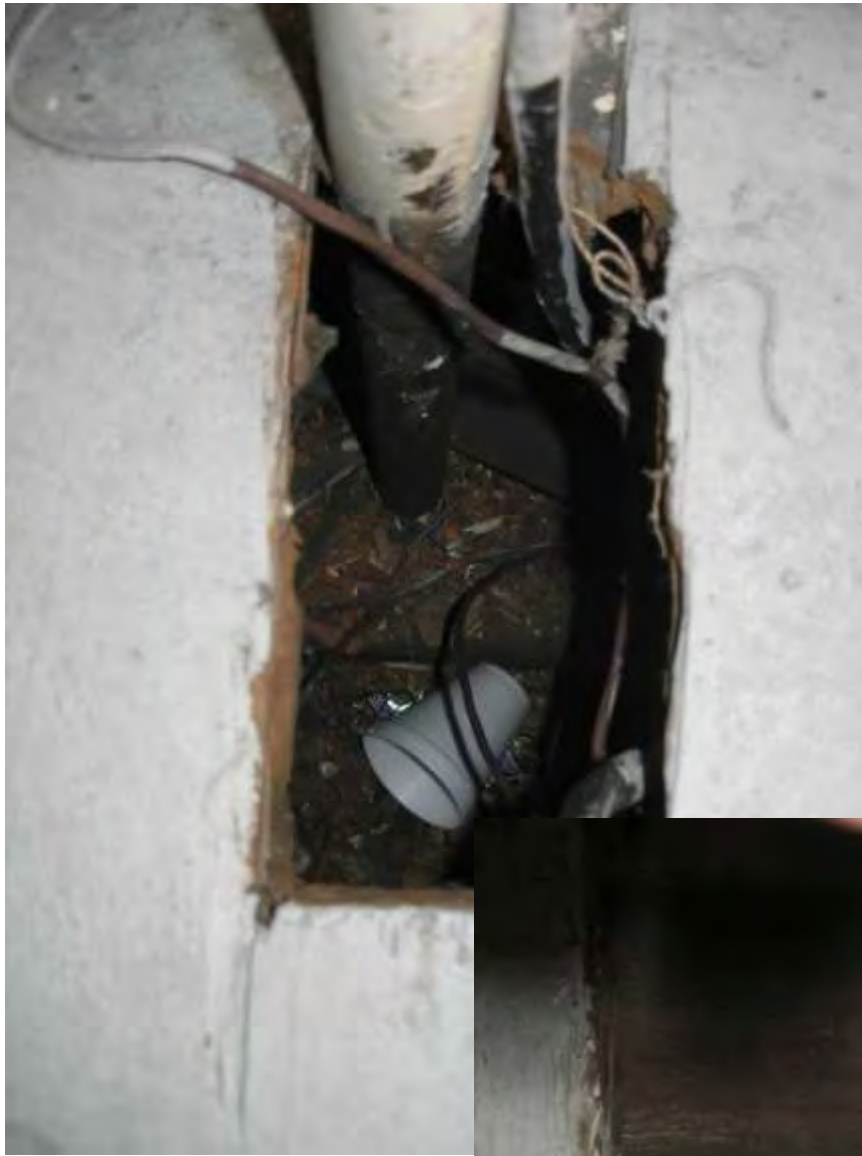
Photo 23. Suspension Rod through Balcony Framing
