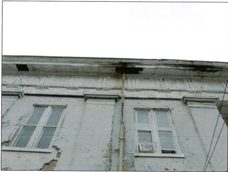
Missing Stucco, Downspout and Peeling Paint
