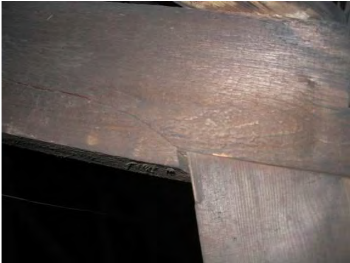
Photo 19. Cracking at Support Notch at Top Chord of Roof Truss
