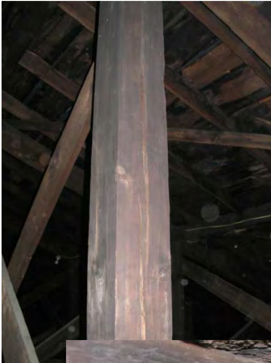
Photo 17. Cracking/Checking in Vertical Timber Post
