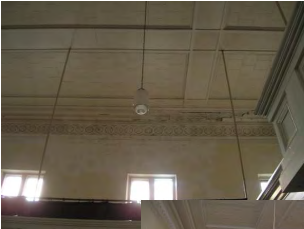
Photo 7. Another View Showing the Balcony Suspension Rods coming through the Ceiling
