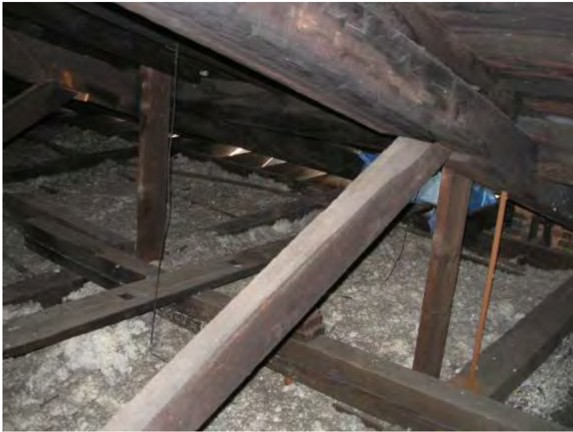
Photo 15. Another view of Roof Trusses Showing Supports for Suspended Balcony
