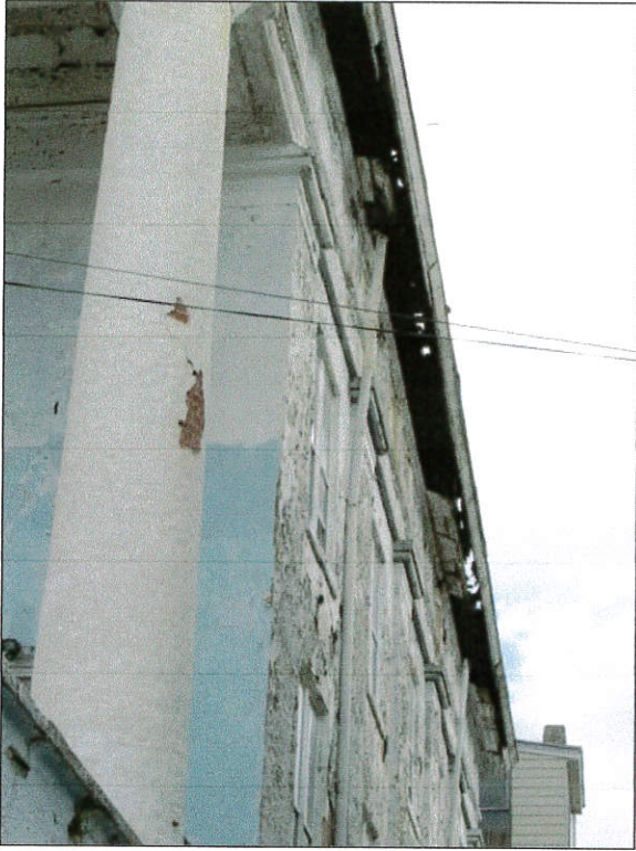
South Side Eave/Missing Column Flutes
