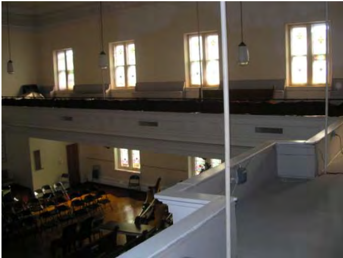
Photo 3. View from the Balcony showing Suspension Rods
