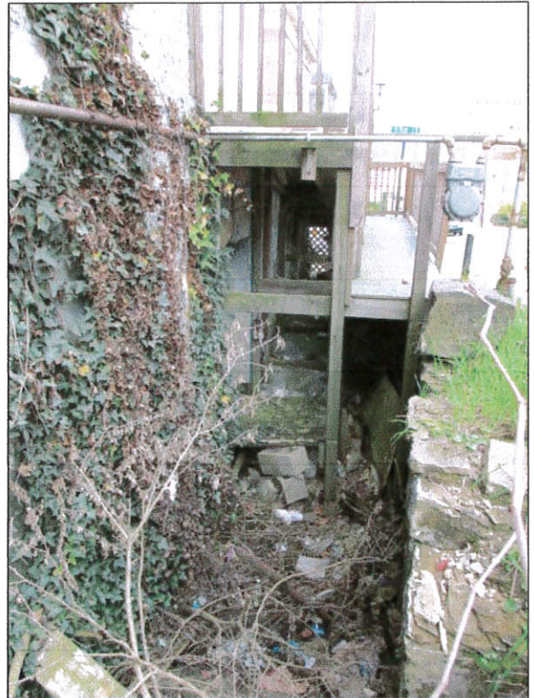
Failed Retaining Wall
