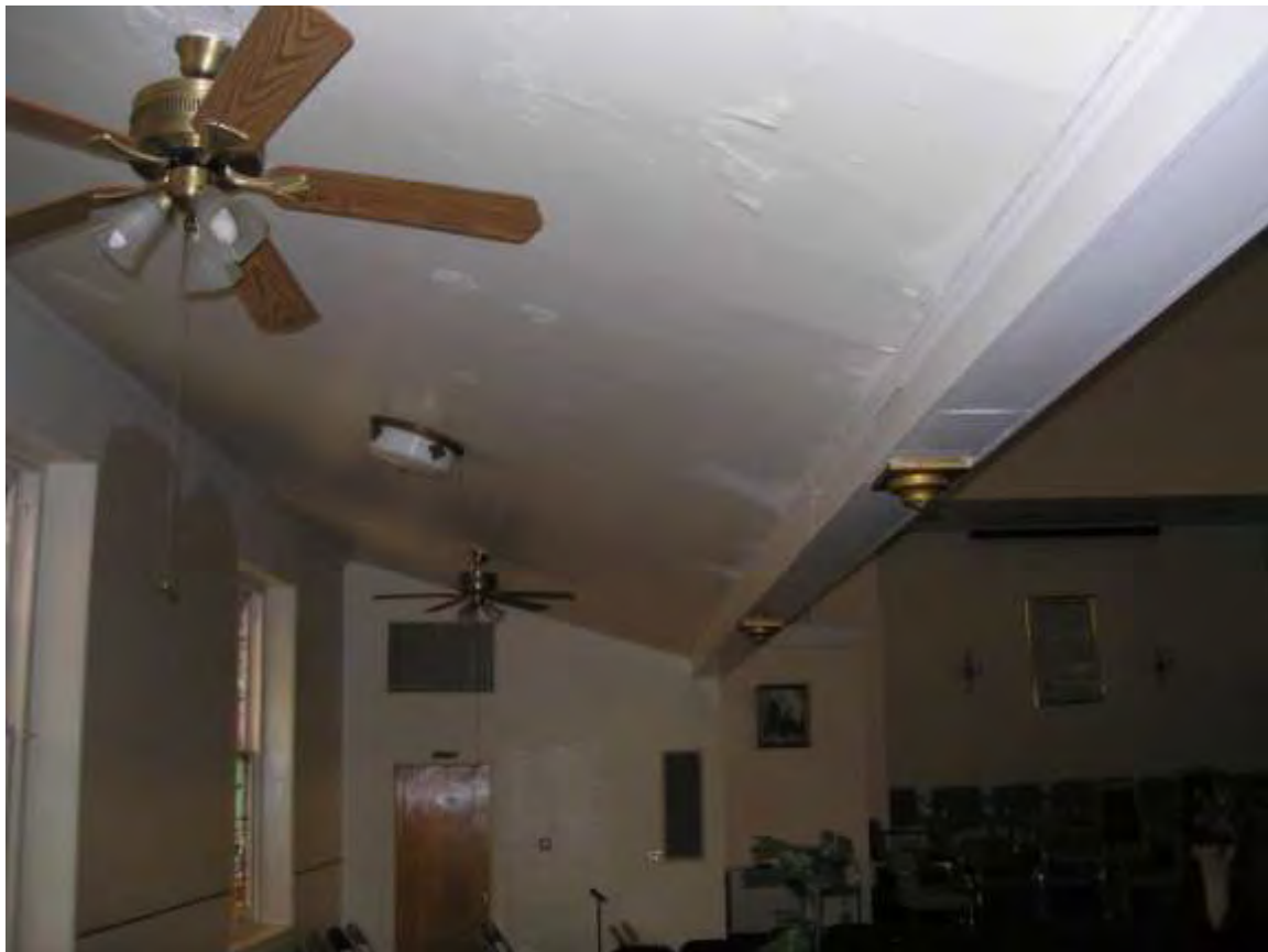
Photo 22. Sloped Ceiling below Balcony Showing Suspension Rod Support Locations
