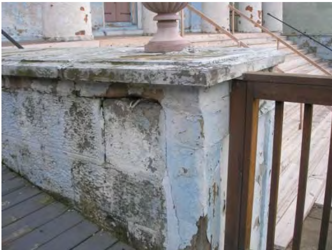
Photo 30. Cheek Wall at North-West Corner of Steps Showing Open Joints
