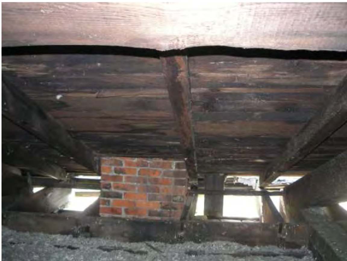
Photo 20. Deterioration of Framing at North Eave
