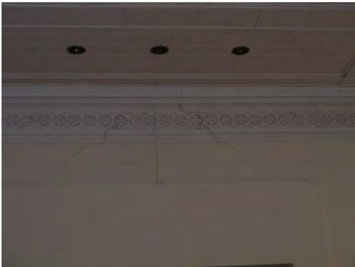
Photo 26. Cracks Above Opening at Front of Church
