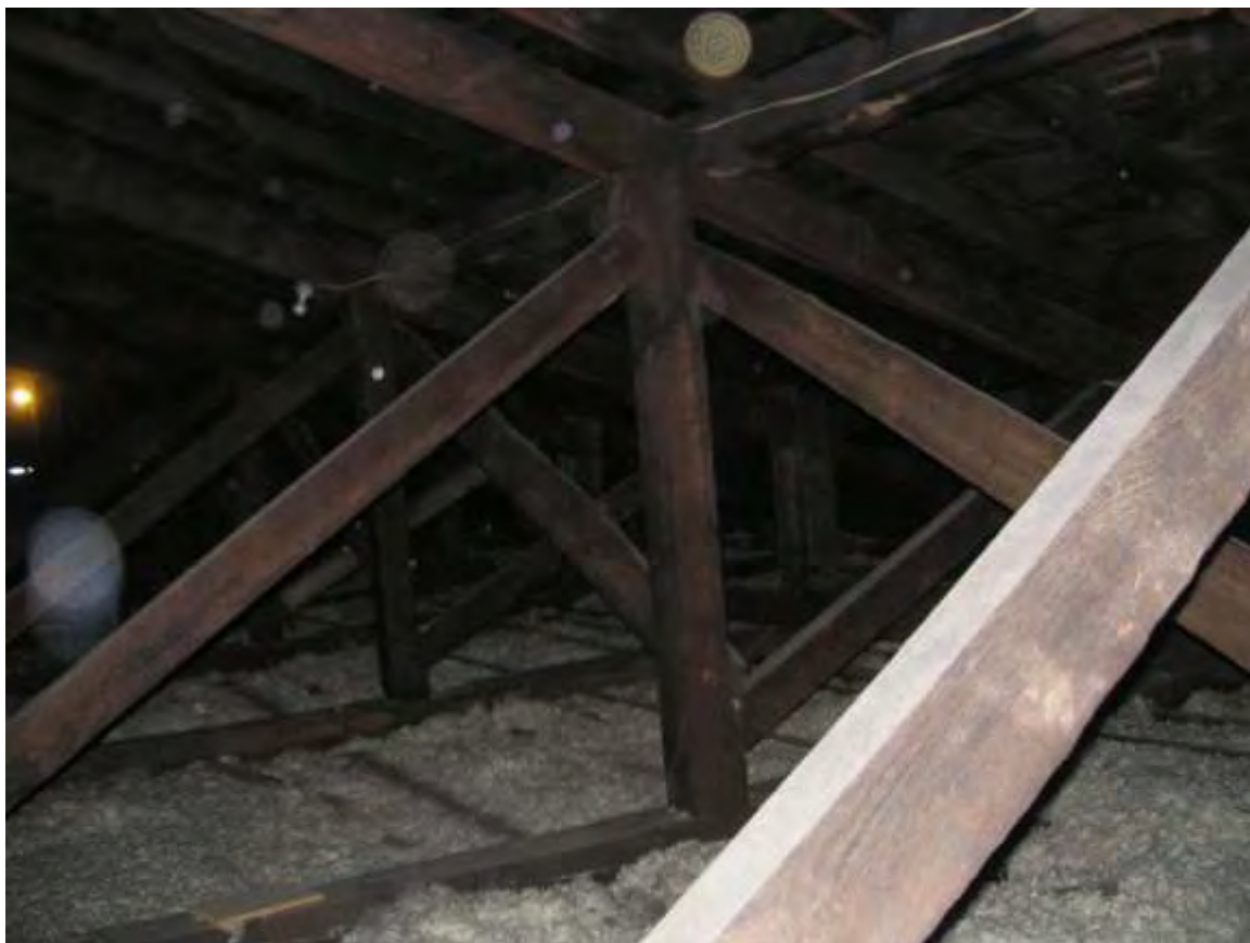
Photo 12. View of Heavy Timber Roof Truss
