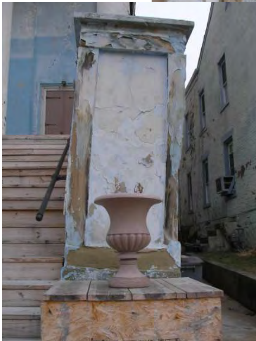
Photo 36. End View of Cheek Wall at South-West Corner of Steps Showing Wall Movement to the Outside
