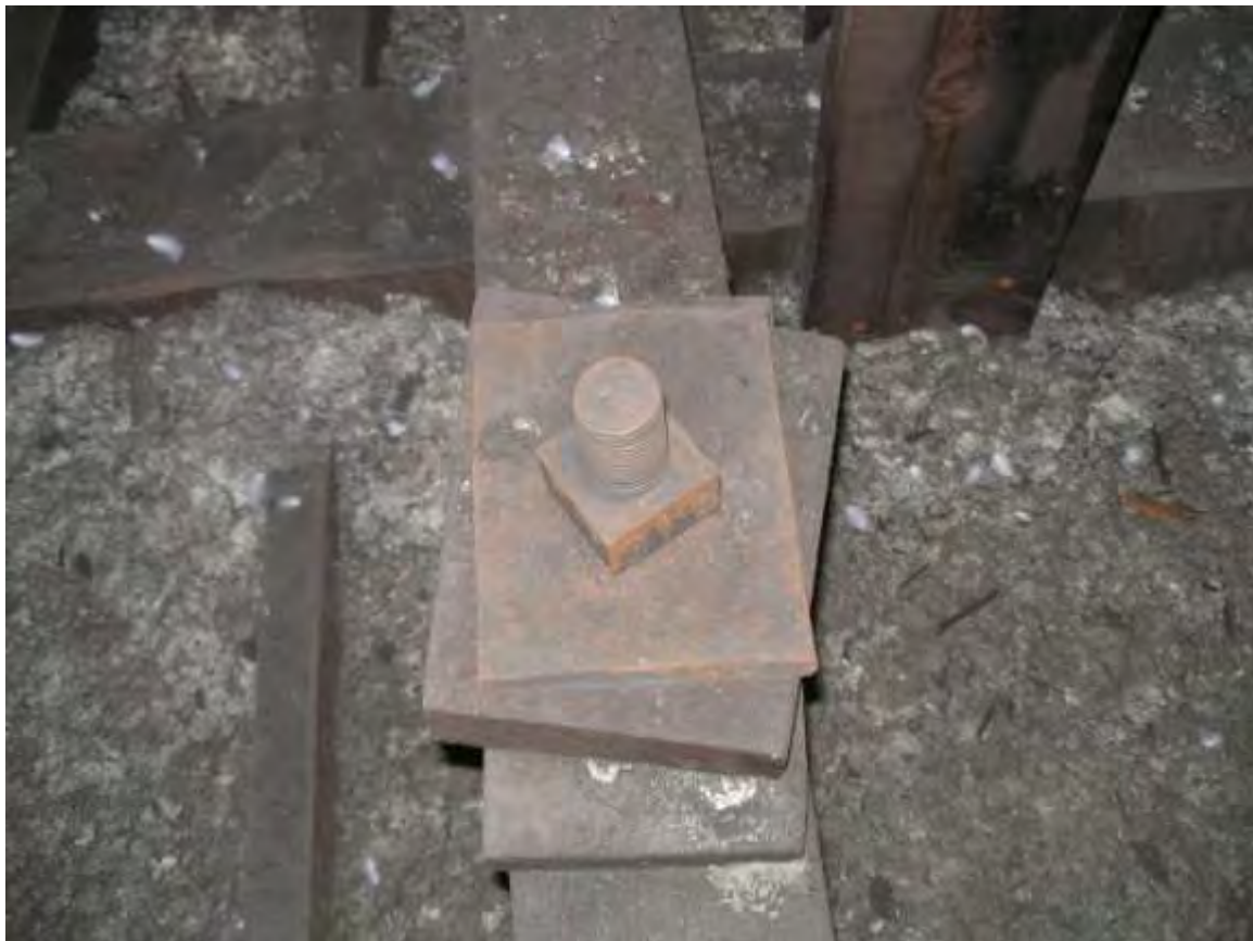
Photo 16. Balcony Suspension Rod Anchorage
