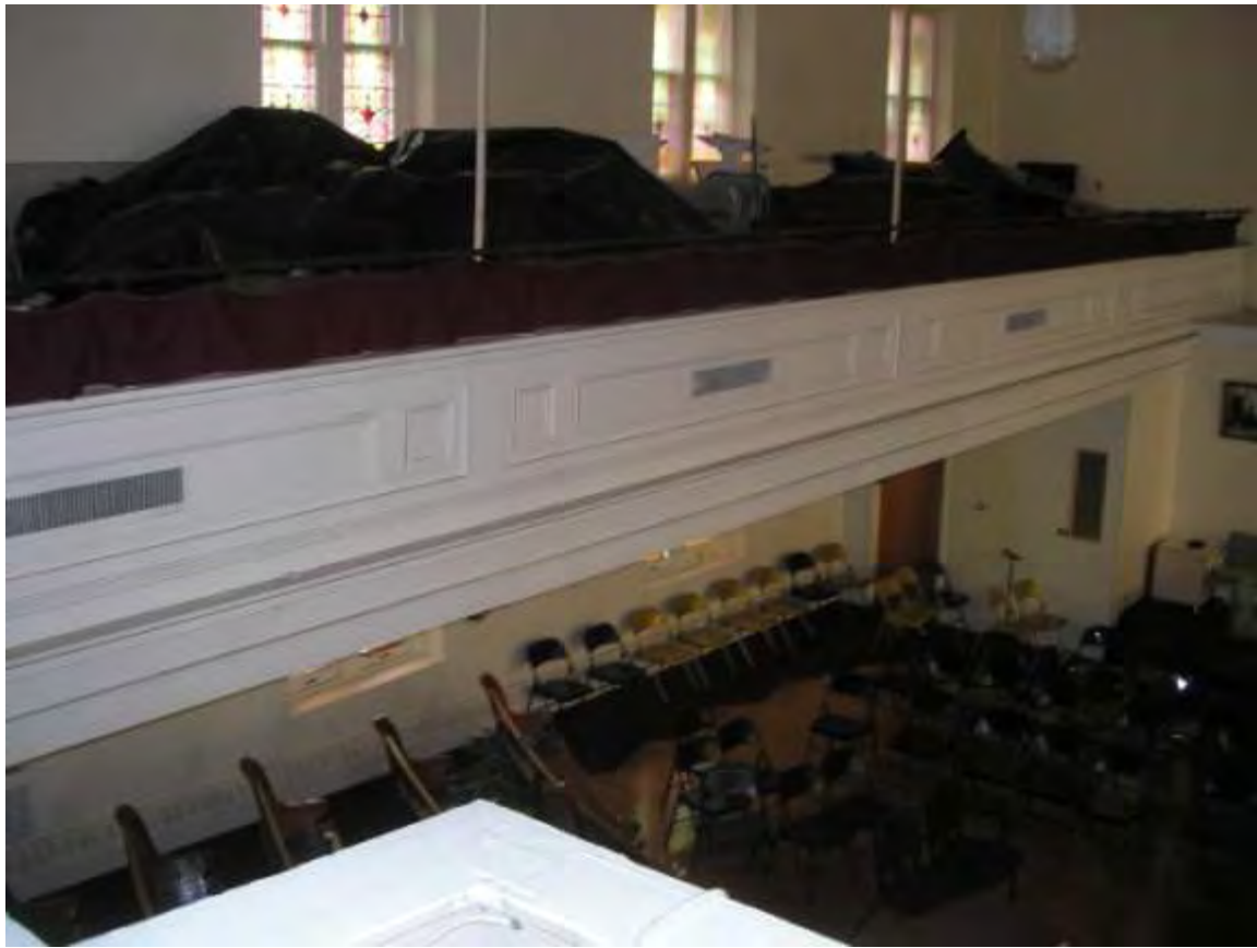
Photo 21. Suspension Rods Supporting Balcony
