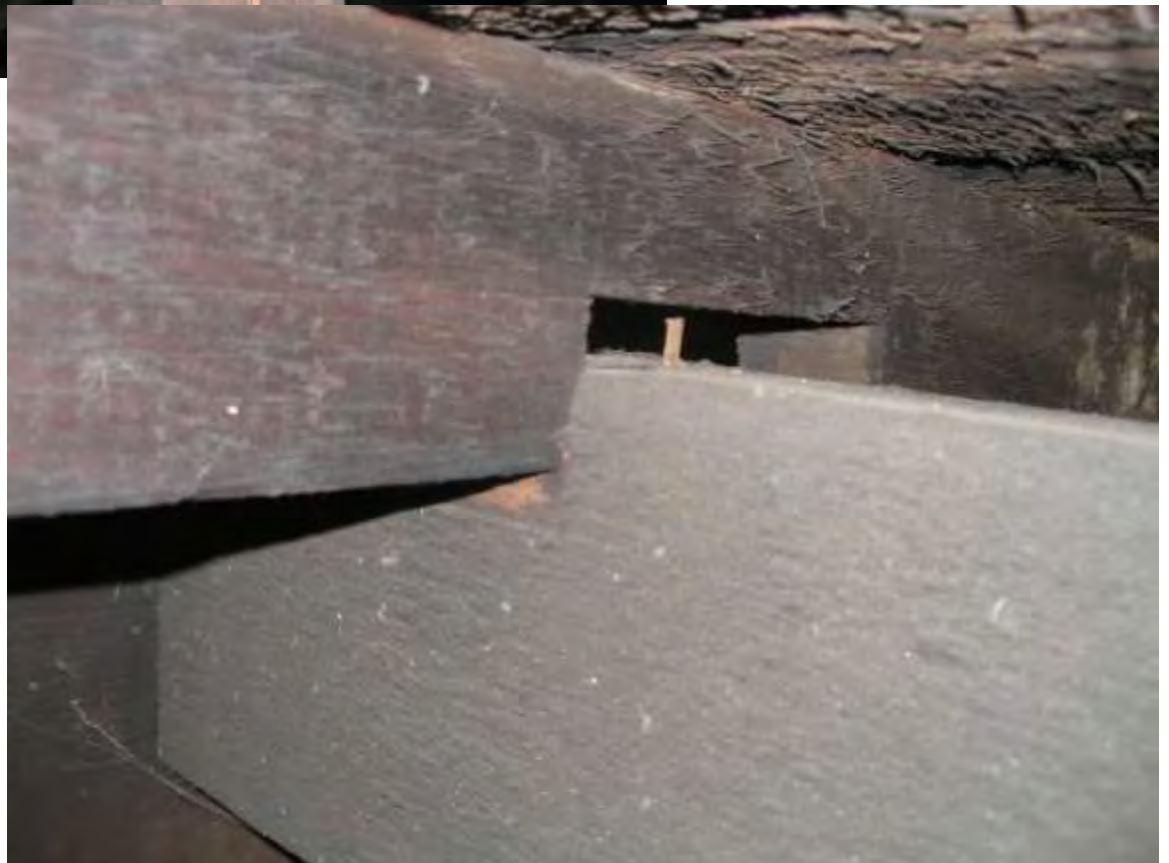
Photo 18. Roof Rafter Lifted Up From Support Beam
